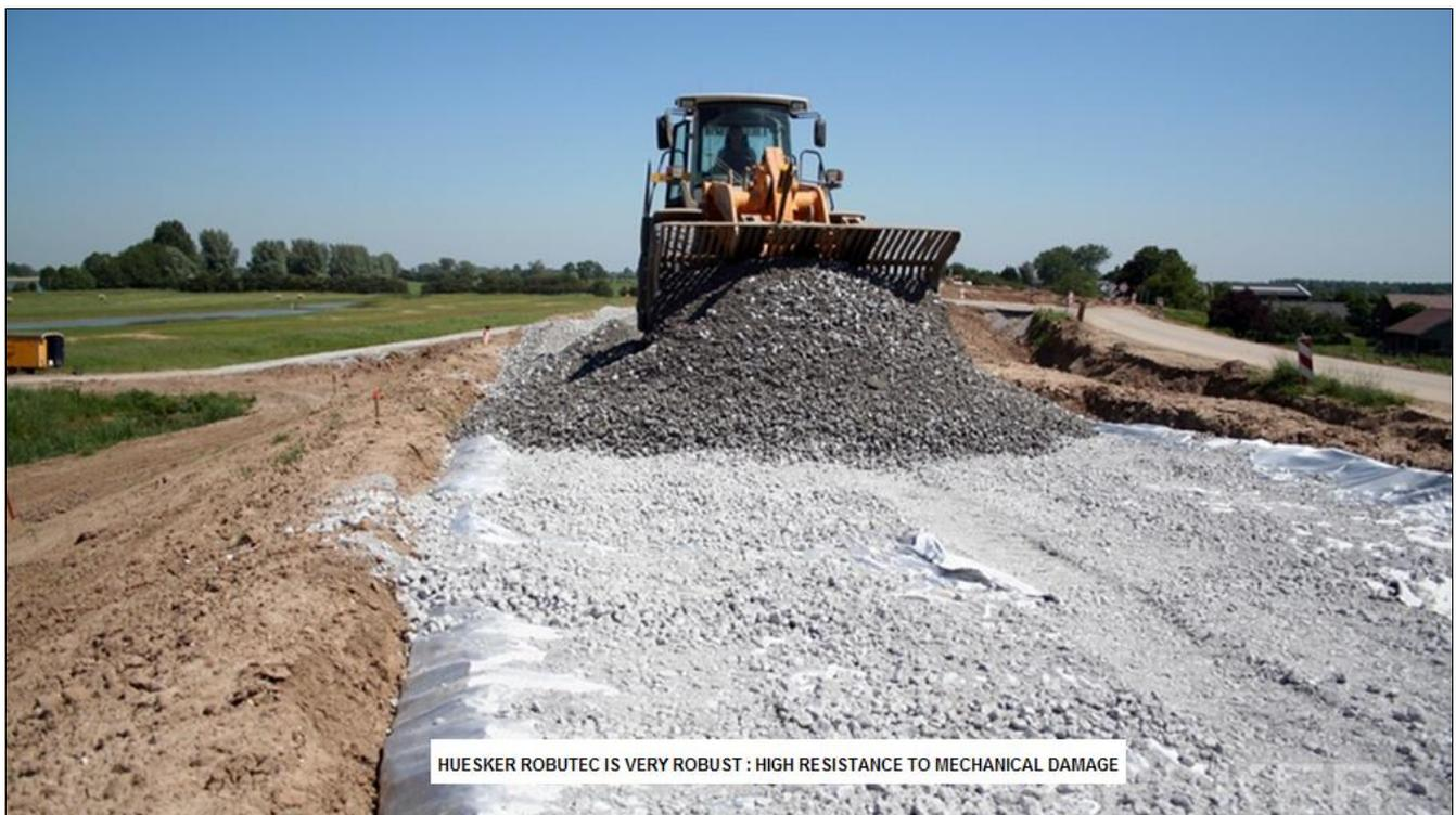
HUESKER ROBUTEC IS VERY ROBUST : HIGH RESISTANCE TO MECHANICAL DAMAGE
