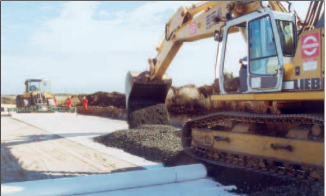
*Forward placement of the stone layer onto pretensioned Stabilenka® 1000/100*
