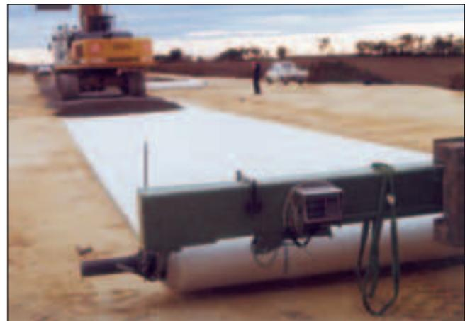
HUESKER's development - a special-purpose device for laying and pre-tensioning **Stabilenka® 1000/100**
