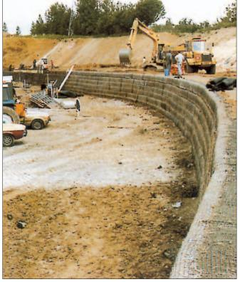
Two Bunds with front slope angles of  $80^\circ$  were built around a supermarket distribution centre to shield the residents of Snodland from the noise of the centre that will be open 24 hours a day.
