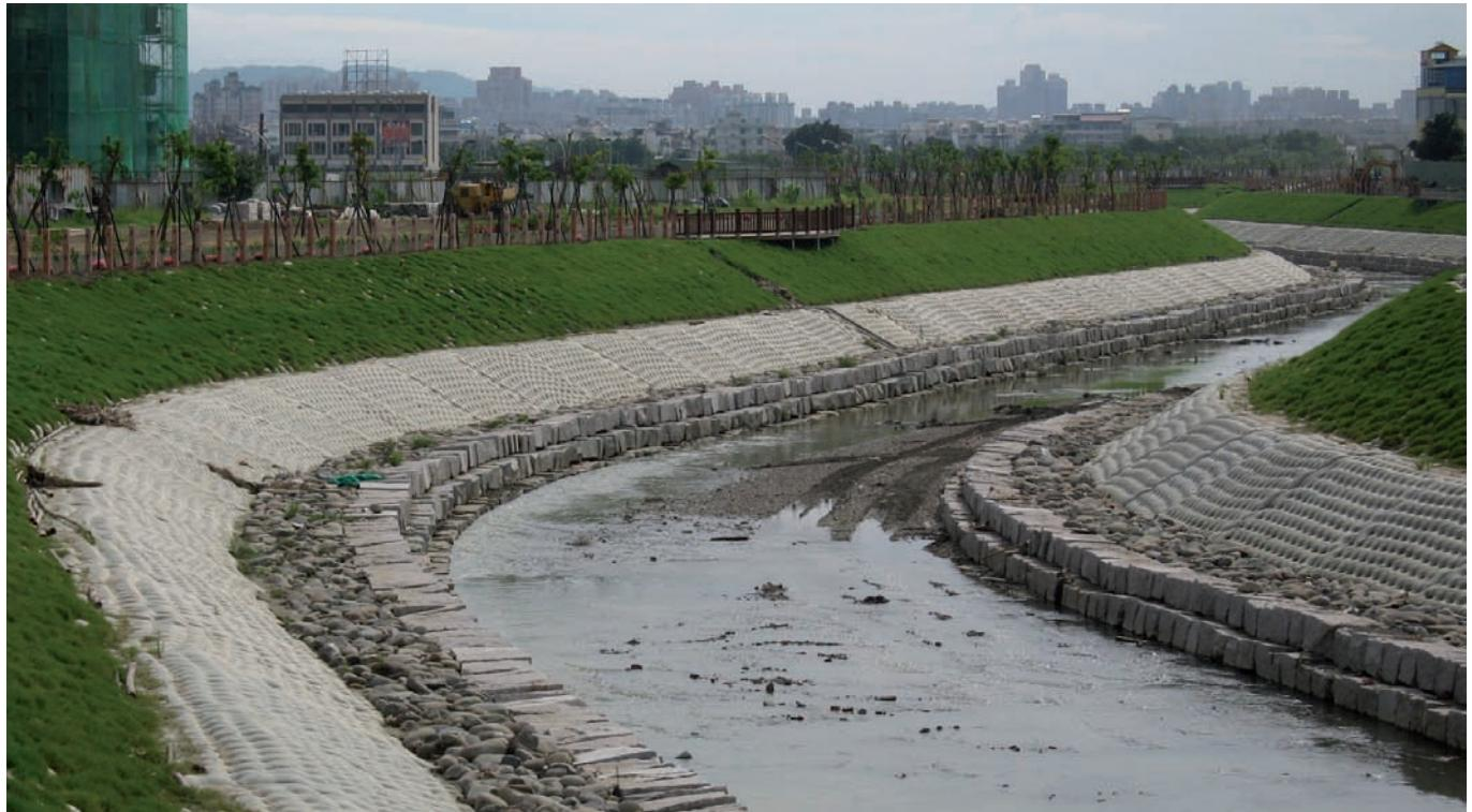
**Incomat®** consists of two high-strength woven geotextile layers connected together with flexible spacers, thereby producing a former which can be filled with concrete. The presence of spacers means that thickness of the **Incomat®** is adjustable to between 6 cm and 60 cm.
