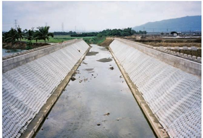
As a revetment, **Incomat®** can be used for dykes, dams, groynes, jetties and breakwaters. As a protective layer or sealing element, **Incomat®** can be used for slurry tanks, rainwater retention basins or fire reservoir ponds. Likewise, **Incomat®** acts as erosion control for overflow routes, dyke openings, inlets and outlets of dyke sluices or flood barriers and stilling basins.
