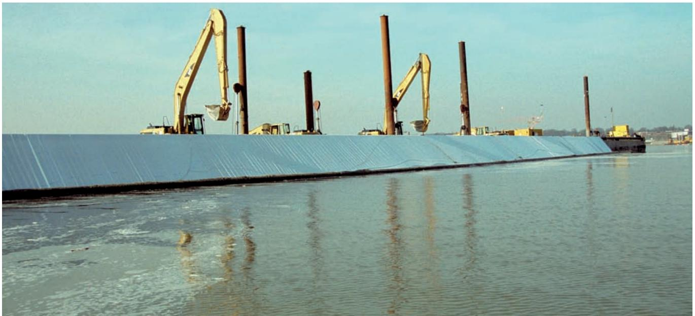
Geotextile reinforcing elements in the foundation base of groynes, breakwaters, dams or dykes are generally required when the sub-soils consist of low-strength cohesive soils.
