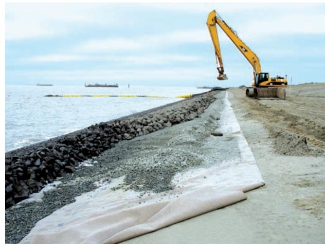
**HaTe®** - nonwoven geotextiles are often used to separate two soil layers of different grain sizes. The properties of a non-woven geotextile can also be varied to provide suitable filtration characteristics.
