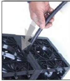
Insert the irrigation tube and cut to size at the ends
