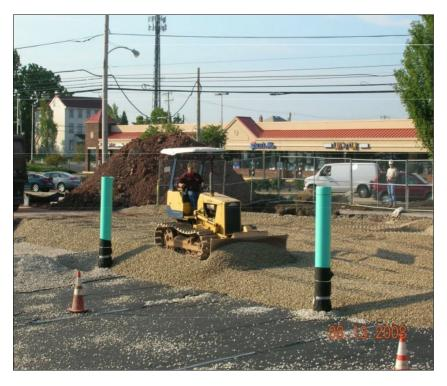
The Atlantis System offers structural strength that enables the application of granular backfill material with a small mechanical shovel. The system also offers inspection points that also serve, if ever required as a cleaning point.
