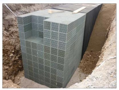
**The challenge:** The construction of HP Data Center involved a total catchment area (including roofs and ground surface) of 21,496 m2, for which HRI Consulting Engineers Ltd would design an infiltration trench that could store stormwater and infiltrate the required volume of water generated by a return period of 10 years in an area of vehicle traffic.
