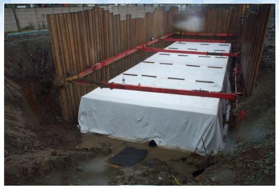
The main offline attenuation tank is made up of single Atlantis Matrix Tank modules with an average cover of 1.10m. The offline attenuation tank has a weir control chamber at the inlet/outlet pipe (225 mm  $\emptyset$ ) to control the runoff into the existing main line stormwater system. The inlet stormwater sewer into the storage control chamber has an oil interceptor. The outlet pipe of 150 mm  $\emptyset$  from the control chamber is connected to the existing stormwater system.
